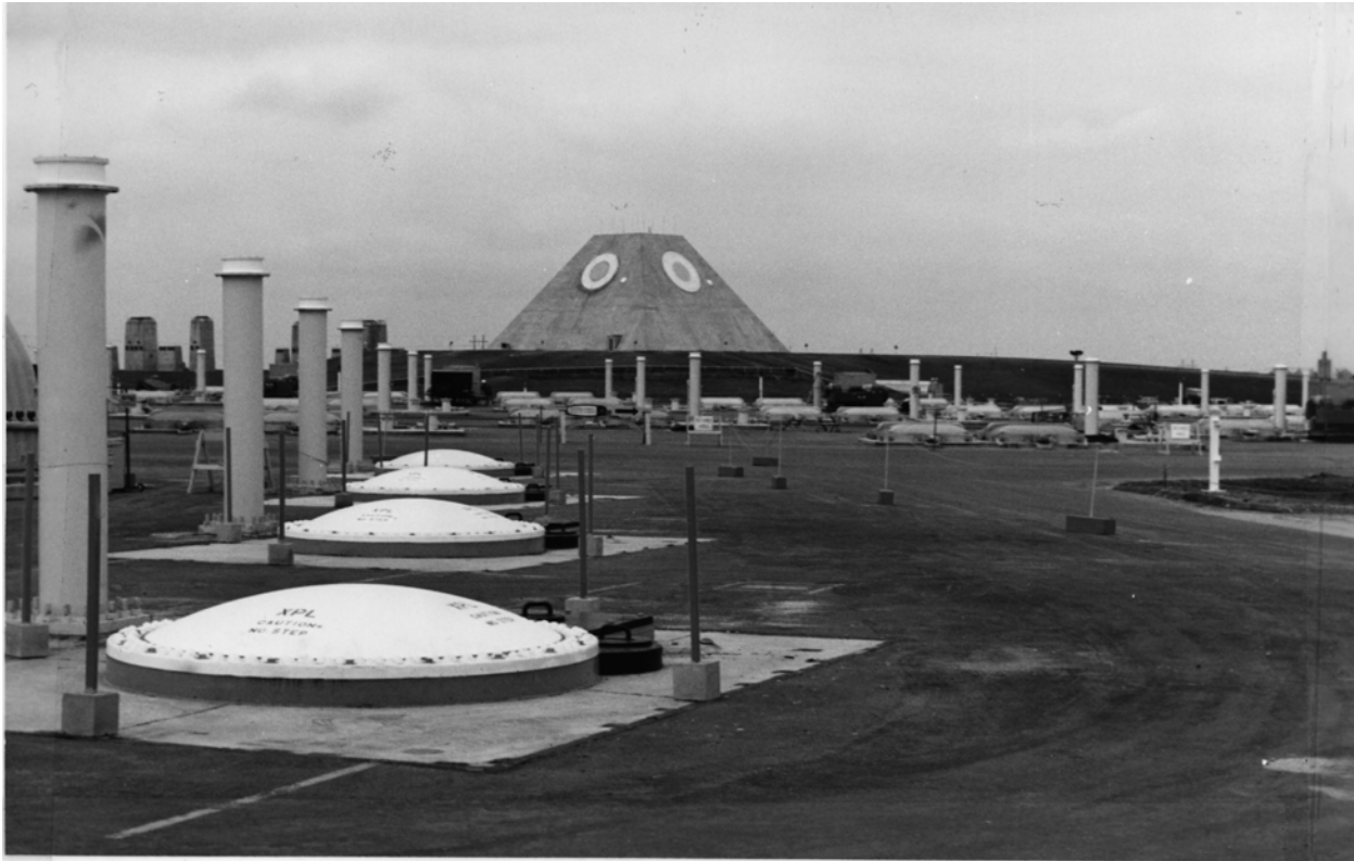
Fig. 2-37. The SAFEGUARD site became the western world's only operational ABM site. The MSR and its missile silos stand ready to protect the nation.
