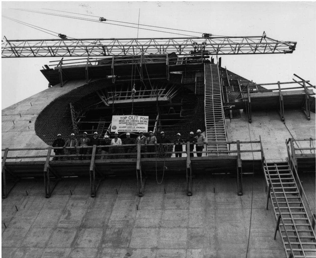
Fig. 2-27. Despite weather conditions, which ranged from -40°F to 100°F, the Top-Out Pour for the Missile Site Control Building took place on 12 October 1971.
